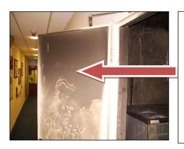
The fire door in this picture demonstrates the effectiveness of a **closed** fire door controlling smoke, heat and fire from spreading.
